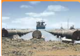
ADCOP SPM & Pipeline Installation
