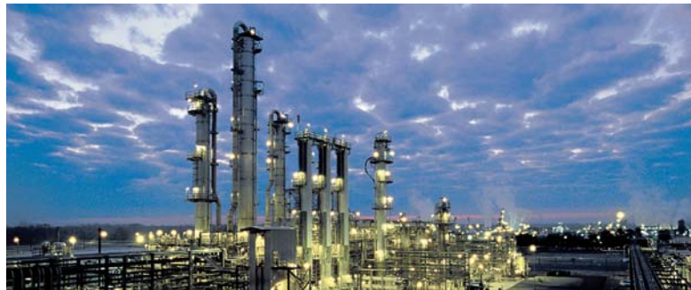
▲ Cutting chemical emissions. This plant produces ethylene oxide/glycols, higher olefins, solvents and 1,3-propanediol (PDO).
