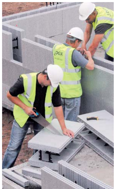
▲ Under construction: Insulated concrete blocks make up this framework.
