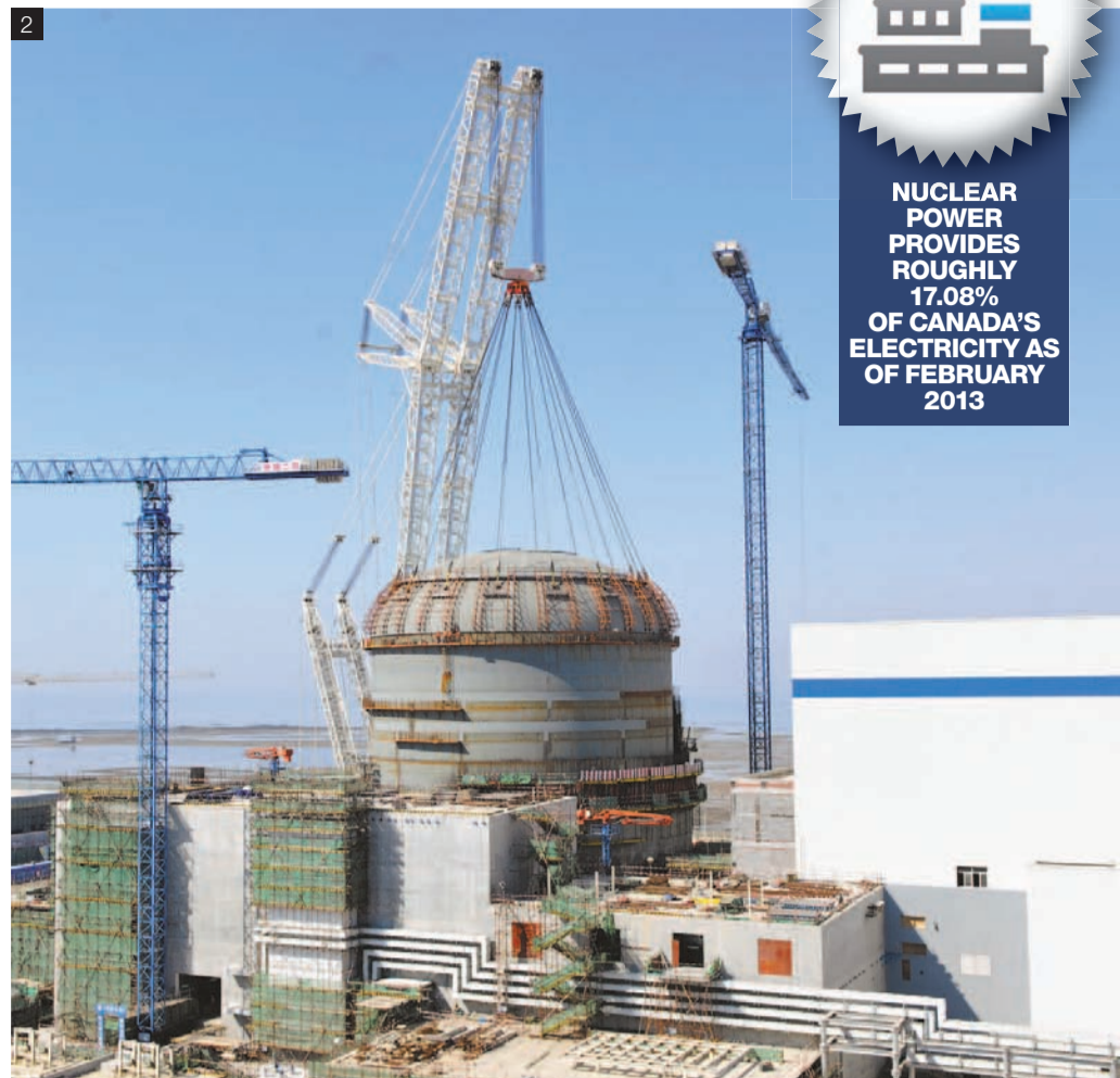
PRESSURIZED WATER REACTORS IN CHINA 1. This plant, located in Qinshan, China is the first nuclear power plant of the country to use Canada's CANDU reactors. PHOTO: CANDU ENERGY INC. 2. Westinghouse AP1000® Pressurized Water Reactor under construction in Haiyang, China. PHOTO: ©2013 SHANDONG NUCLEAR POWER COMPANY LIMITED. ALL RIGHTS RESERVED.
